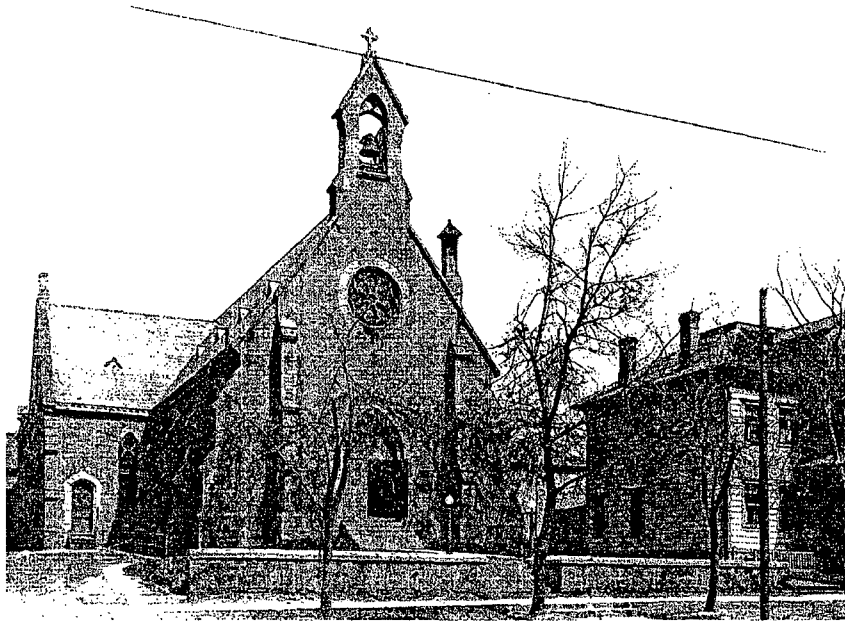
Figure 11: St. Mark's Cathedral Church, c. 1880
