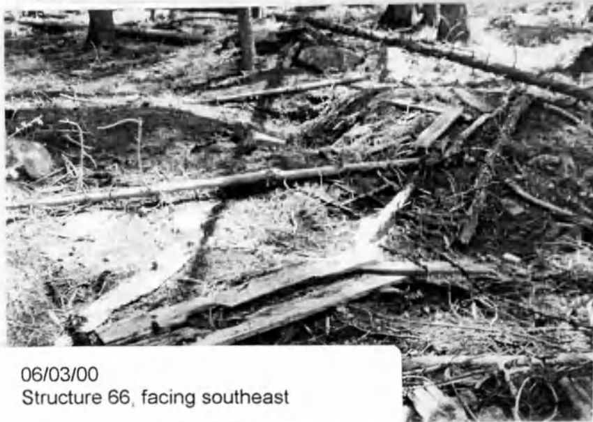
06/03/00 Structure 66, facing southeast
