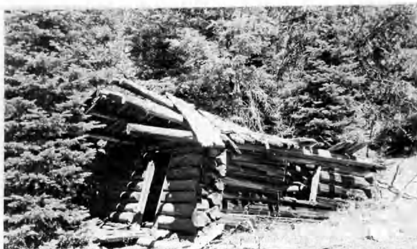
06/03/00 Structure 83, facing northeast
