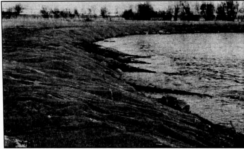
Figure 2. Placement of log bars to deflect the erosive force of the current away from the bank and toward the center of the channel.
