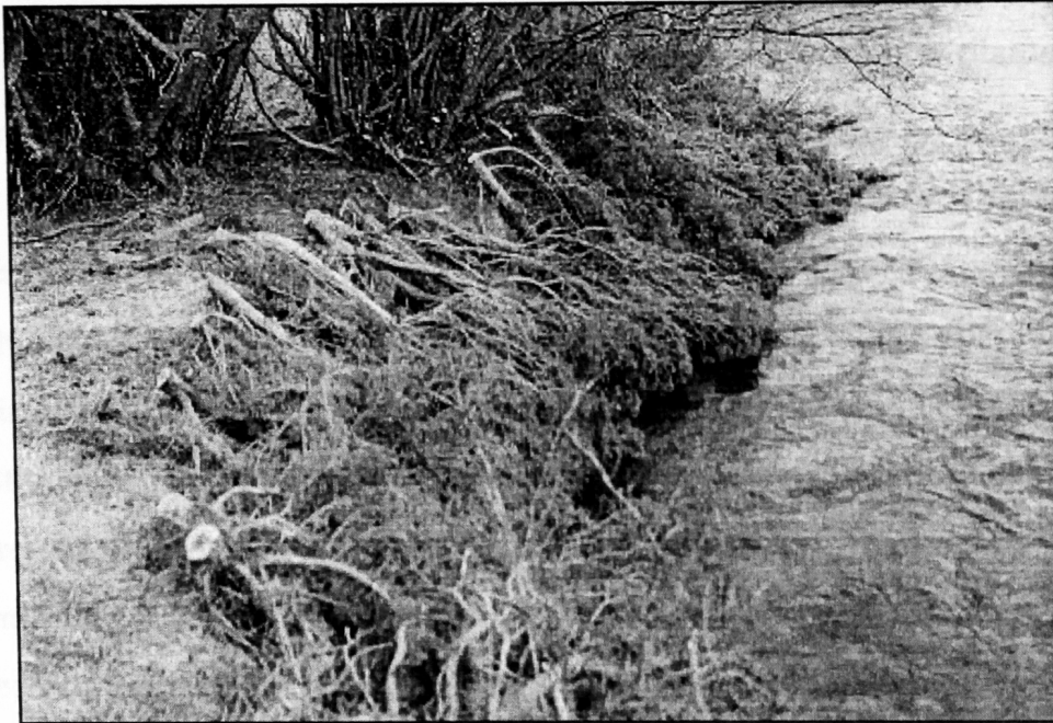
Figure 4. Placement of Juniperus scopulorum (Rocky Mountain juniper) revetments along the outer edge of a vertical bank. The revetments are designed to reduce the erosive force of the current and to minimize the impact of winter ice floes.
