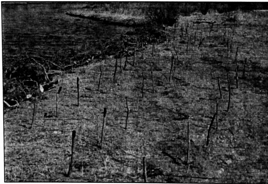
Figure 5. The vertical Salix spp. cutting planting method. Cuttings extend approximately 30 cm (1 ft) above the bank surface.
