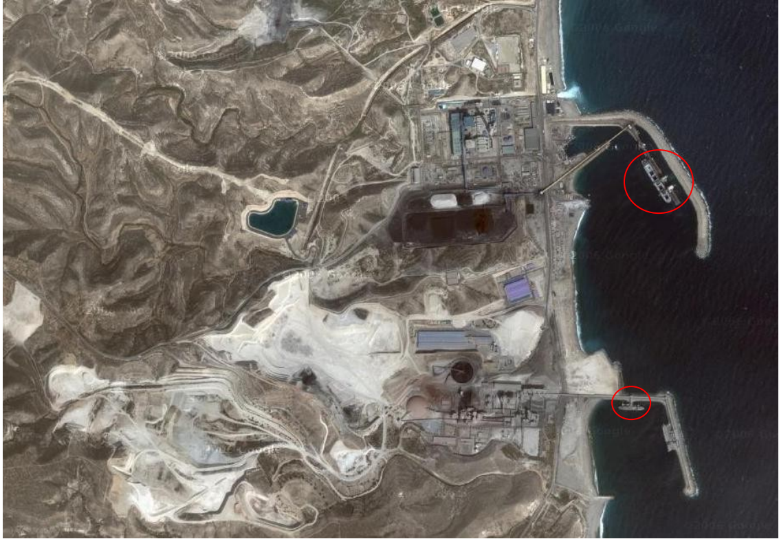
FIGURE 16 Europe's biggest desalination plant located near Carboneras, Almería. The red circles identify two large tanker boats docked at the facility to offer a scale comparison. (Source: http://maps.google.com )
