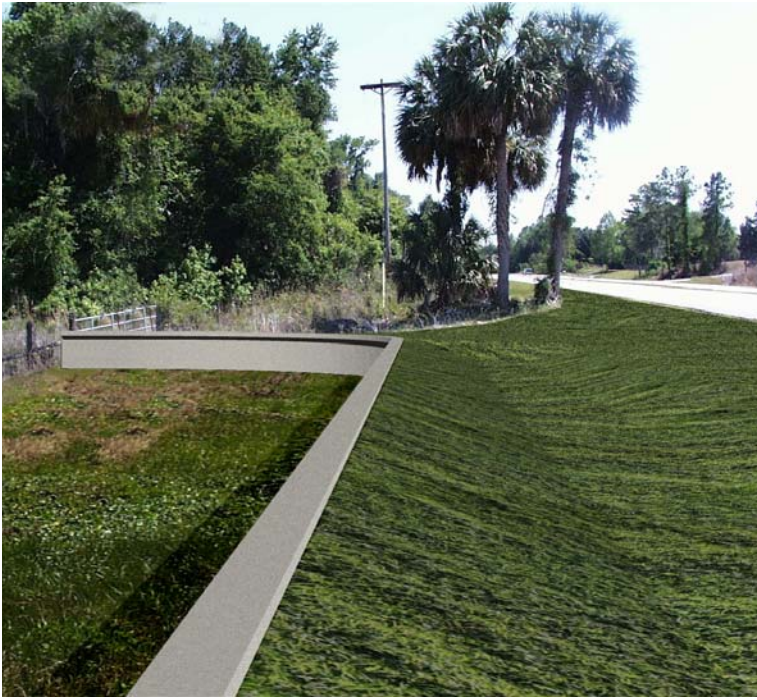
Figure A-8. Paynes Prairie Ecopassage – Artist rendition. Concrete wall with lip. (Florida). Photo: D. Forsyth.
