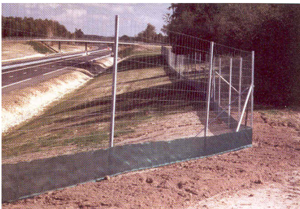
Figure A-1. Wire fence with plastic fabric mesh (France). Photo: Bank et al. 2002. Figure A-2. Wire fence with smaller mesh at the bottom. Photo: Bank et al. 2002.
