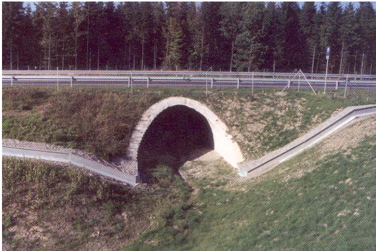
Figure A-12. Example of a combination of barrier methods. Arched culvert with large fence along highway and metal rail for amphibians and reptiles (Germany). Photo: Bank et al. 2002.
