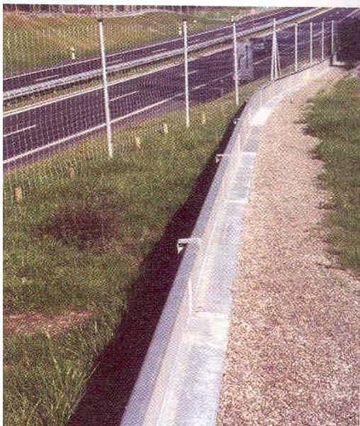
Figure A-5. Galvanized steel rail with lip for amphibians and reptiles (Germany). Photo: Bank et al. 2002.
