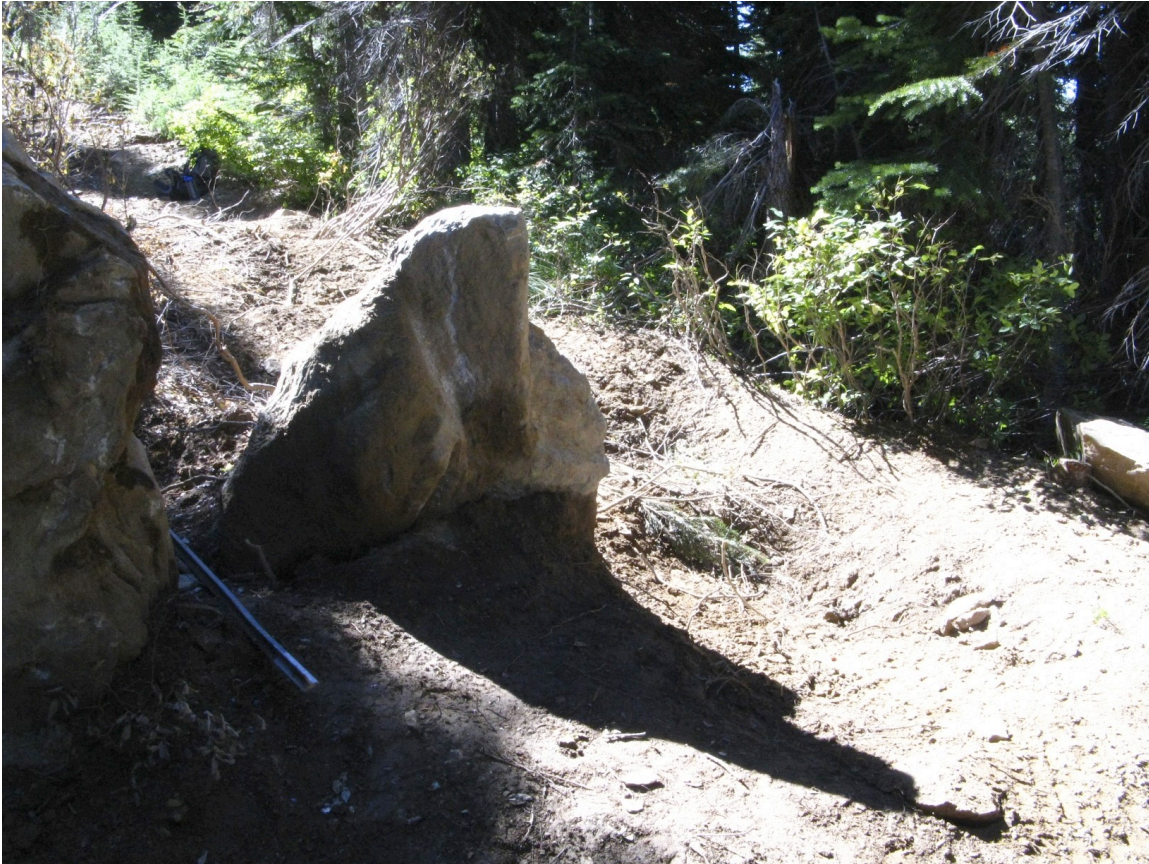
Users removed a boulder (far right) and informational sign to gain motorized access to the restored route (Copper Ridge)
