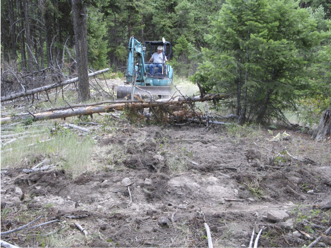
Decompaction, Erosion Control, and Slash Application (Chimney Rock)
