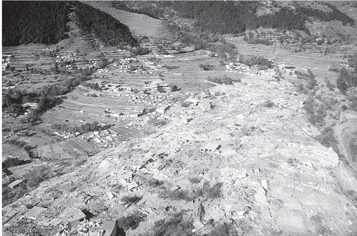
FIGURE 1 The population of Balakot in the North-West Frontier Province was particularly vulnerable to the 8 October 2005 earthquake. A significant proportion of the damage to this urban area was attributed to the siting of structures on the active fault as well as to the lack of seismically appropriate engineering methods and poor quality construction. (Photo by L. Owen, November 2005)
