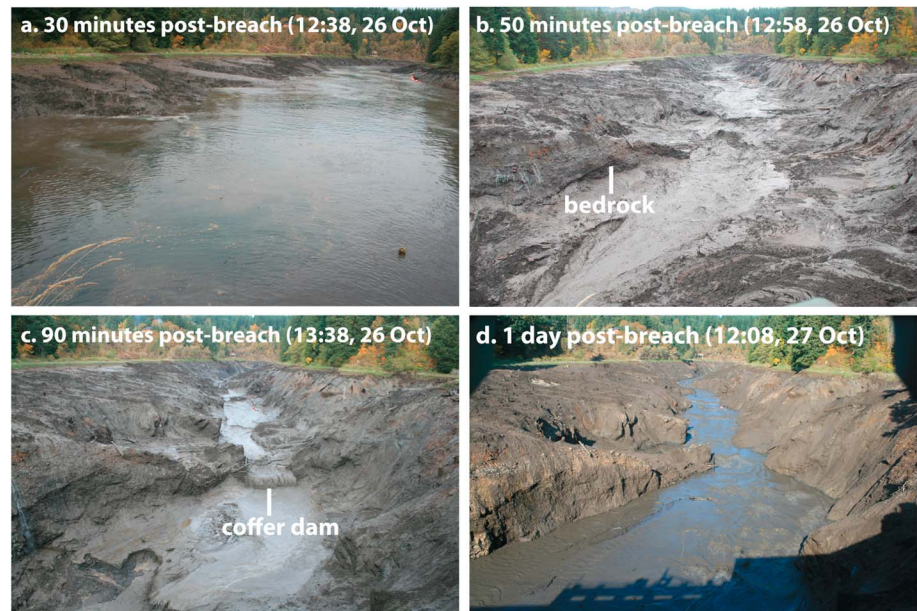
Figure 3. Time series of reservoir drainage; images taken from dam crest facing upstream show lower ~600 m of former Northwestern Lake. (a) Reservoir water-surface elevation has declined by 10 m, and slump scars indicate onset of landslides; (b) mass failures, exposed bedrock, and slurry in channel; (c) mass failures have slowed, and incision has exposed coffer dam; an estimated 160,000 \text{ m}^3 of erosion has occurred in the visible reach as of this time; and (d) side slopes show little change relative to Figure 3c, eroded material from farther upstream in transport. Videos of time-lapse imagery from this camera station are provided in the supporting information.
