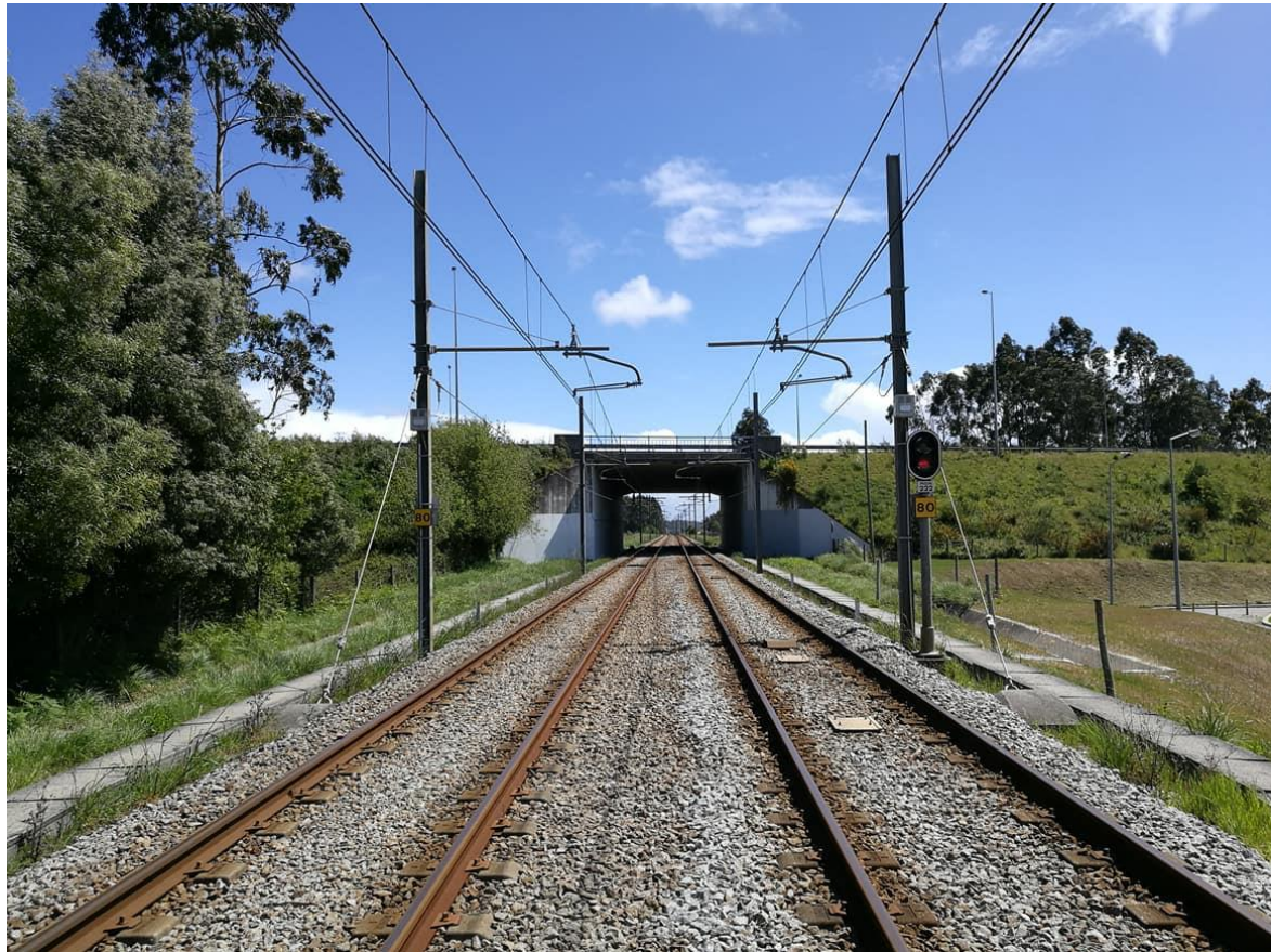
FIG. 1. Single mast structure supporting OHLE
