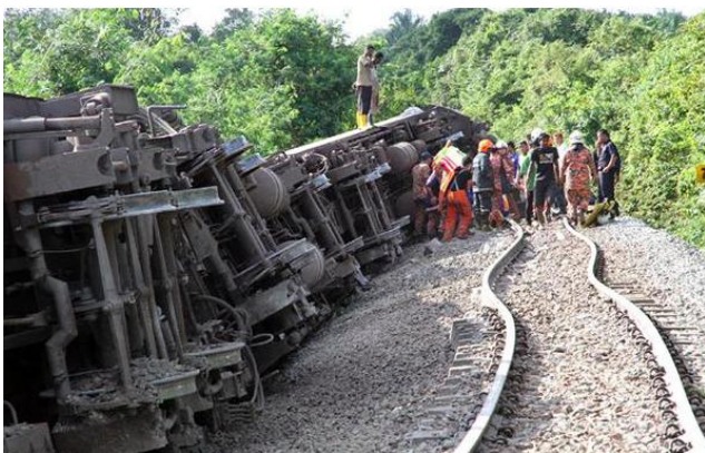
Figure 10: KTMB train derailed due to rail buckling and had landed on its side, trapping the driver and injuring about five passengers just before the Kempas, Johor station southern part of Malaysia
