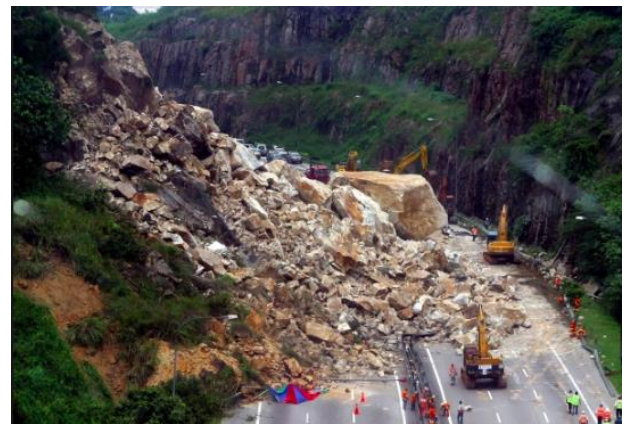
Figure 8: The Bukit Lanjan rockfall along the New Klang Valley Expressway, in November 2003, resulted in a six month closure of that particular stretch
