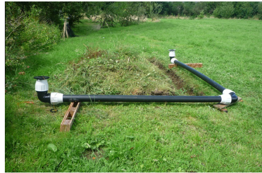
Fig. 4. Pipe rig just prior to burial.
