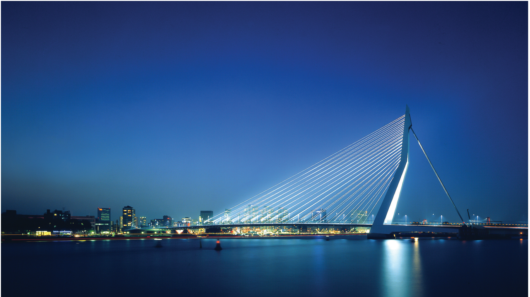
Erasmus Bridge, Photo by Christian Richters
