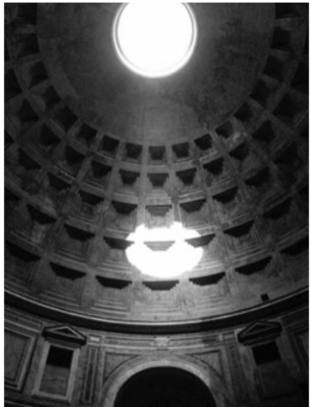
Figure 3. A harmony of mood and atmosphere The Roman Pantheon (Rome), completed by the Emperor Hadrian about 126 AD. Here the architect made the world's largest unreinforced concrete dome. The diameter of the inscribed plan and dimension to the oculus and are the same 142 ft.
