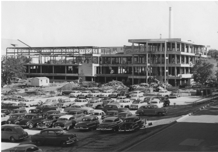
Union under construction
