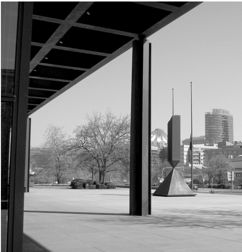
Figure 6. Ludwig Mies van der Rohe, Neue Nationalgalerie, Berlin, 1968 . Detail of the pin connection with the Richard Serra sculpture in the background.
