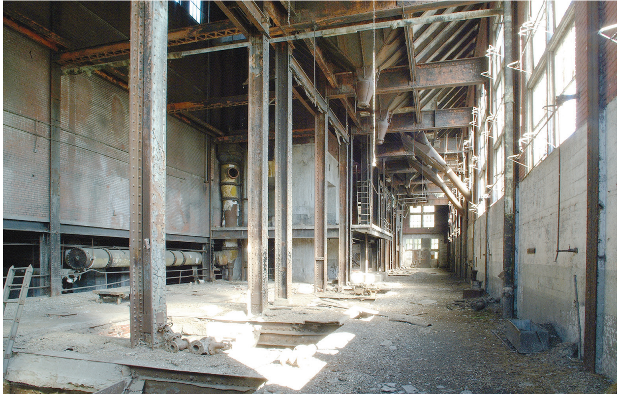
Figure 4. Powerhouse Existing Conditions
