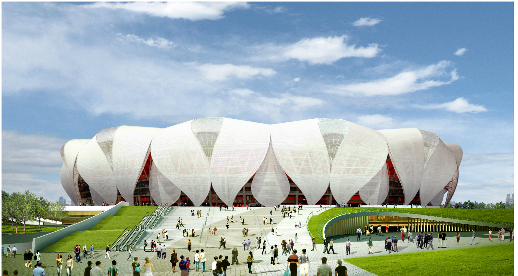
Fig. 5. The Hangzhou stadium. The stadium will have 80,000 seats and is under construction. The project will be completed in 2013.
