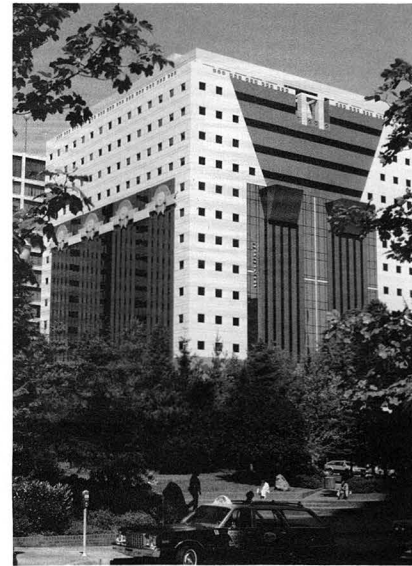
The Portland Building, Portland, Oregon. Michael Graves. 1979-83.
