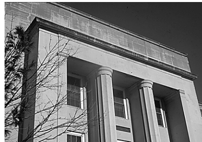
Fig. 14. Skidmore Owings and Merrill, School of Engineering, University of Maryland, College Park, MD, 1948–52. Photo Schumacher
