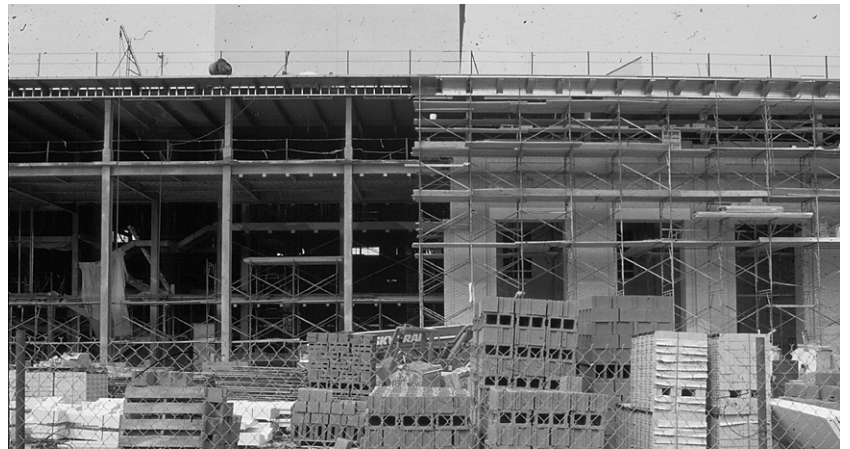
Fig. 17. Purnell Center, CMU, Michael Dennis and Associates, construction photo. Photo Schumacher
