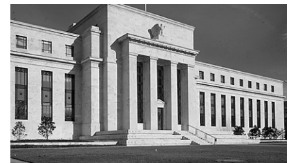
Fig. 4. Federal Reserve Bank, Washington, DC, Paul Cret, 1937. Photo Schumacher
