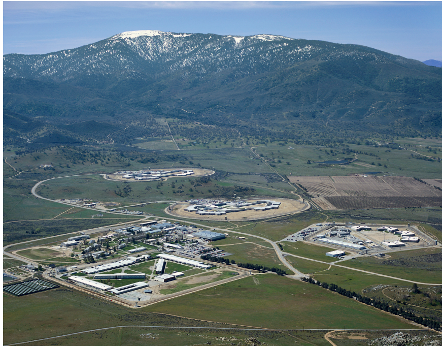
Figure 6. Aerial view of California Correctional Institution [Digital image]. (n.d.). Retrieved from: http://www.cdcr.ca.gov/Facilities_Locator/CCI.html . Used with permission.
