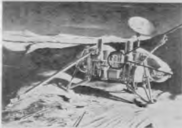
FIG. 1. Position of the biology instrument in the Viking Lander.
