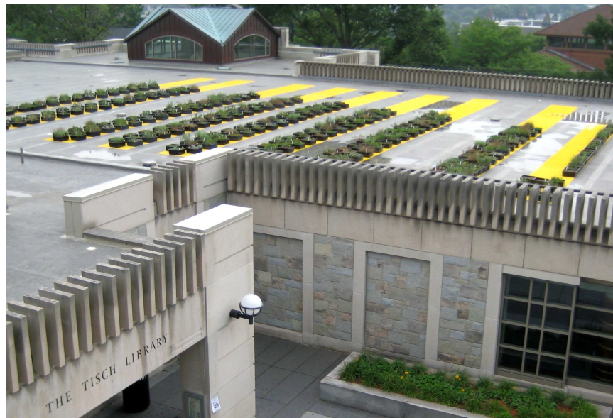
Figure 4. Experimental modular green roof on Tisch Library at Tufts University Medford, MA
