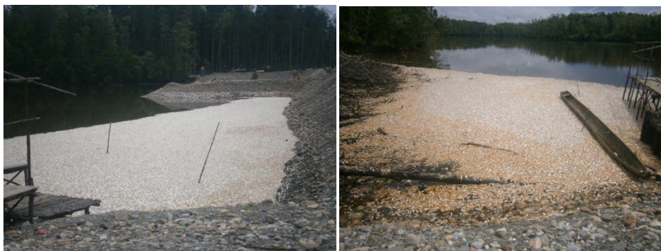
Figure 2. Condition of MME at the west tailing levee on 8 April 2016 (Photo collection of Environment Department of PT. Freeport).
