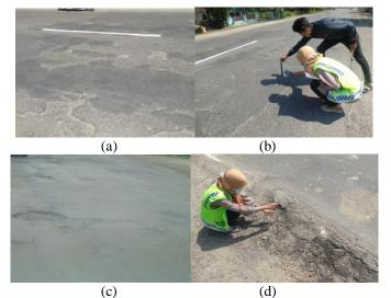
Fig. 2. Road condition identification: (a) Cracking, (b) Rutting (c), Pothole (d) Deformation.
