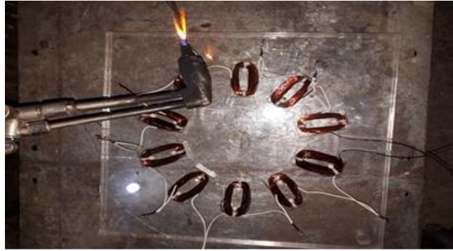
Fig. 11 The winding to the stator installed permanently.
