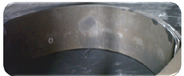
Gambar 3. Plate Liner Eksisting (Lembaran)
