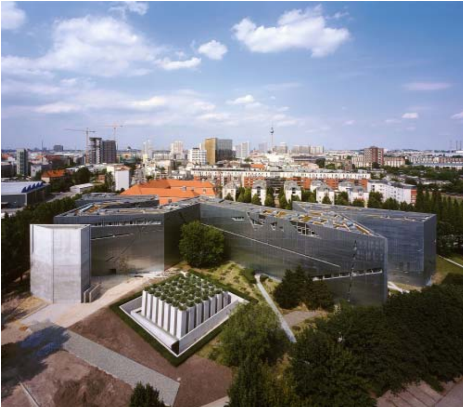
Fig. 2. Daniel Libeskind, Jewish Museum Berlin, City View, foreground center, E.T.A. Hoffmann 'Garden of Exile,' foreground left, 'Holocaust Tower', photo © Bitter+Bred
