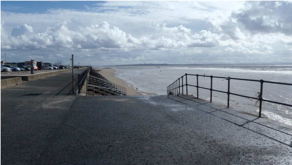
Fig. 2. The Crosby sea wall frontage.
