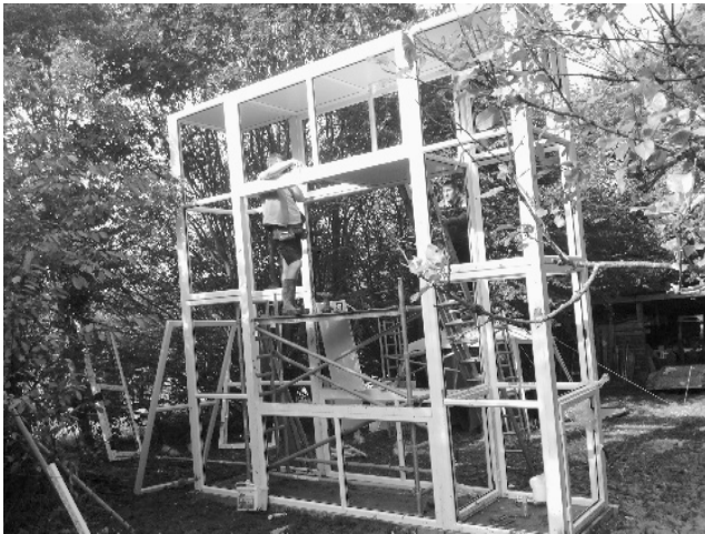
Figure 2. The structure under construction. Source: Bunyard.
