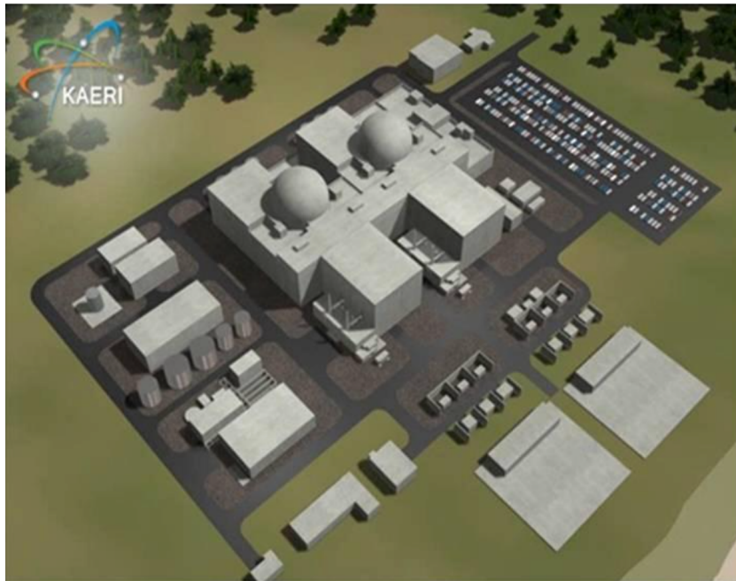
Figure A.I.11. Plan view of the SMART (KAERI, Republic of Korea) twin SMR reactor facility [162] with a net power output of 200 MWe ( 2 \times 100 MWe units).
