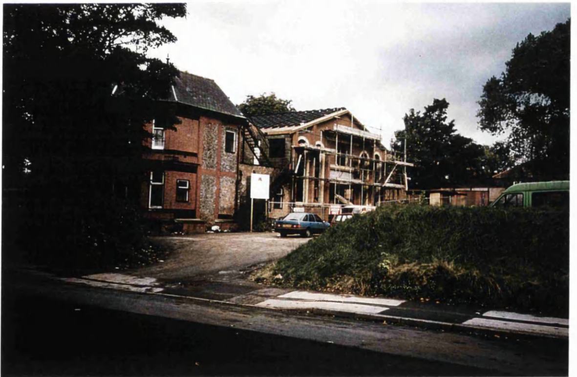
Plate 6.4: Satmar shteible on Northumberland Street (note the building is in the process of being extended: another indication of the growth of the community).
