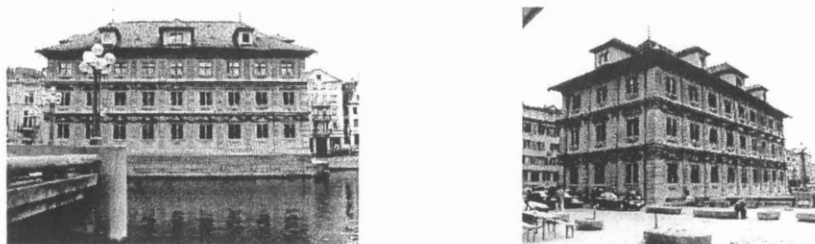
Figure 6.7 Images of the Zurich City Hall from St1 and St3
