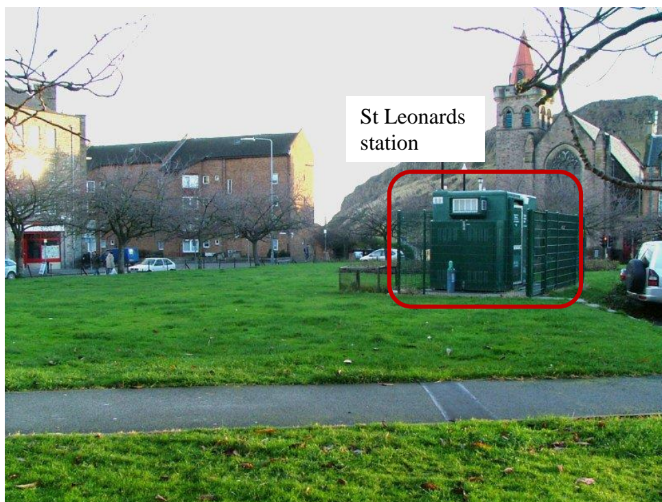
Figure 4.1 Siting of the St Leonards station with respect to the surrounding environment.
