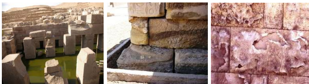
Fig. 1. Forms of physical deterioration affecting some Egyptian monuments resulted from the effects of salinity water
