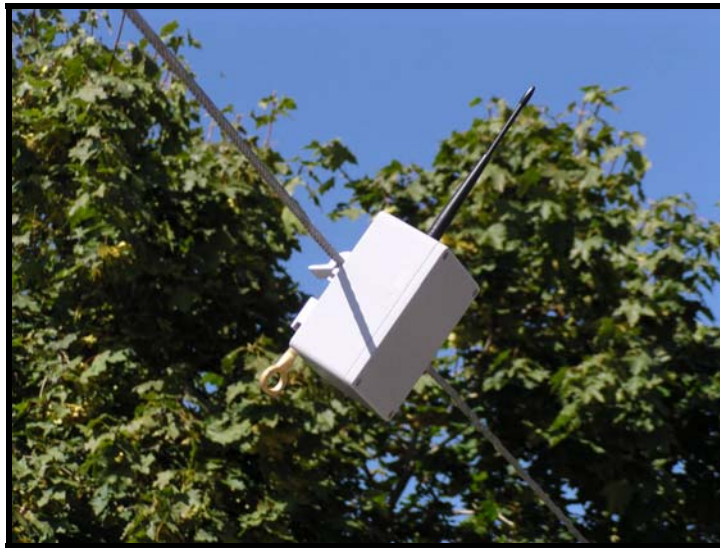
Figure 2. BSI sensor installed on a wire
