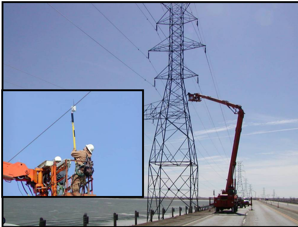
Figure 7. Installation of BSI sensors using a bucket truck and hot stick
