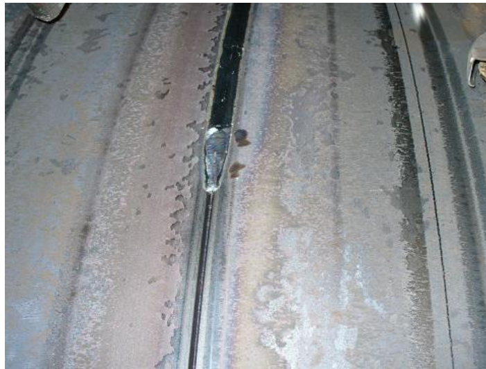
Figure 1.13: External welding of spiral welded pipe [NPC]
