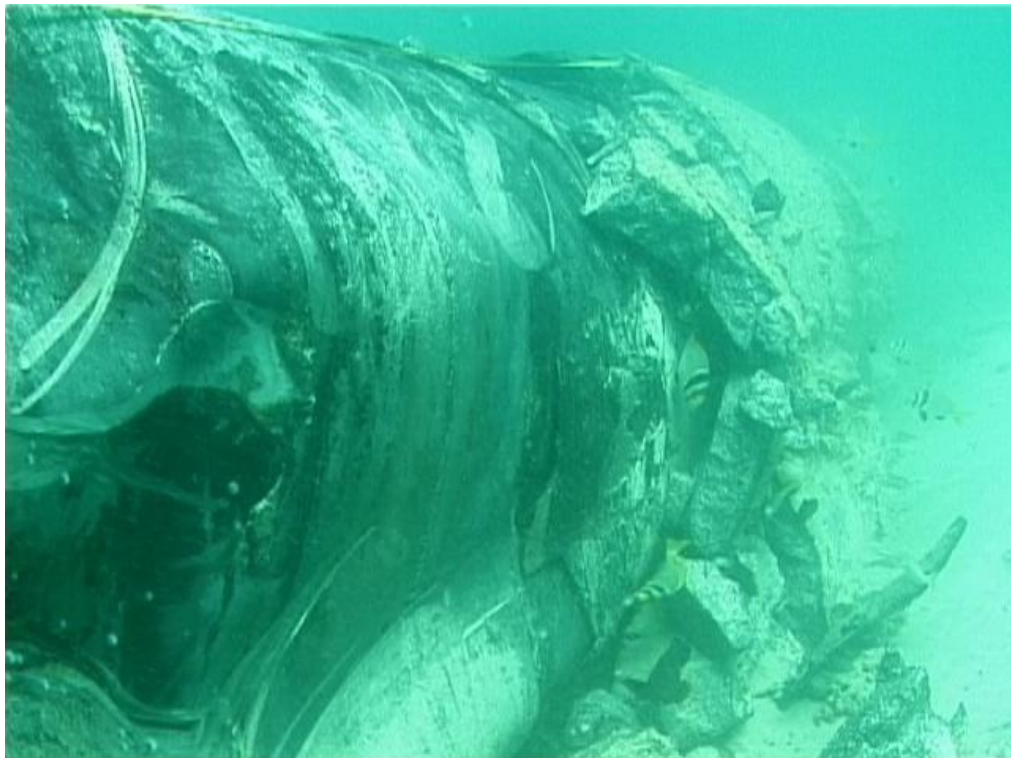
Figure 1.2. Mechanical damage in offshore pipeline
