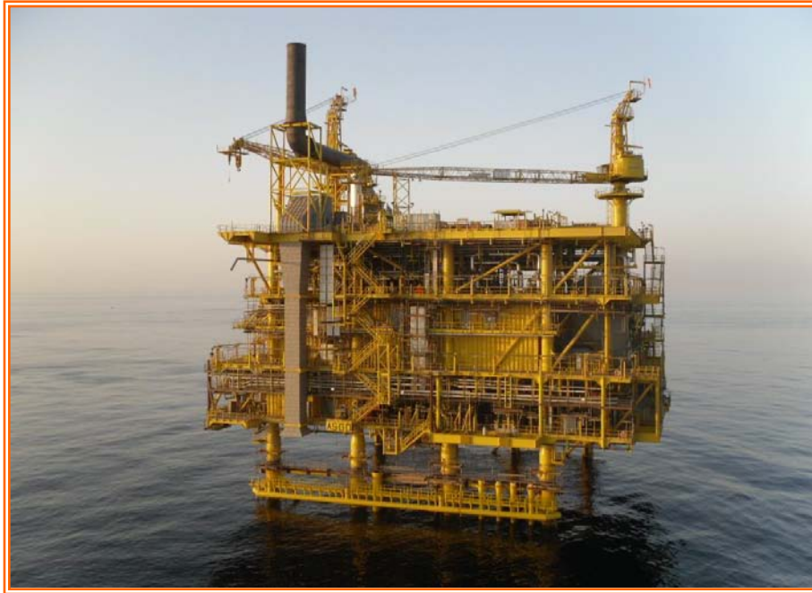
1. Figure 1.1: Offshore Platform (Al-Shaheen Field,Qatar)
