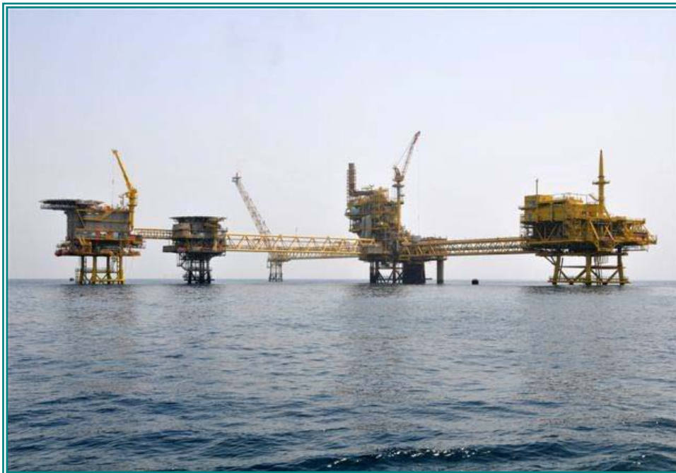
Figure 1.2: Offshore Platform (Al-Shaheen Field,Qatar)
