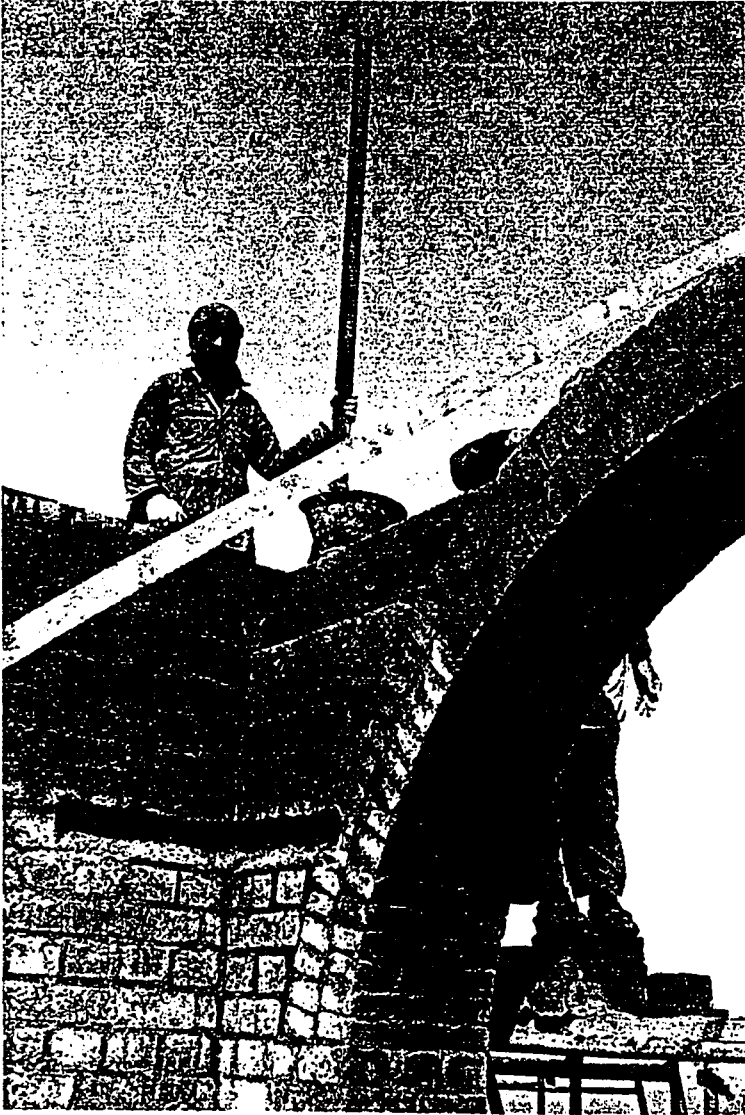
Figure 2.7 Example construction of Exhibit-Centre at Janadria, Riyadh - work above the arch.
