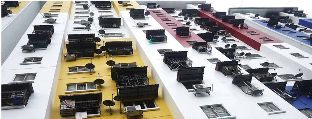
Figure 1. High-rise social housing in Kuala Lumpur.
