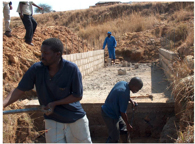
Fig. 6. Constructing the H-Flume in the Potshini catchment.
