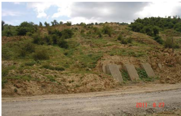
Fig. 5. Lapoş Valley Landslide
