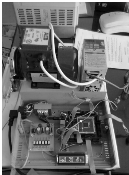
Figure 9. Experimental module of on-line speed and braking control of induction motors
