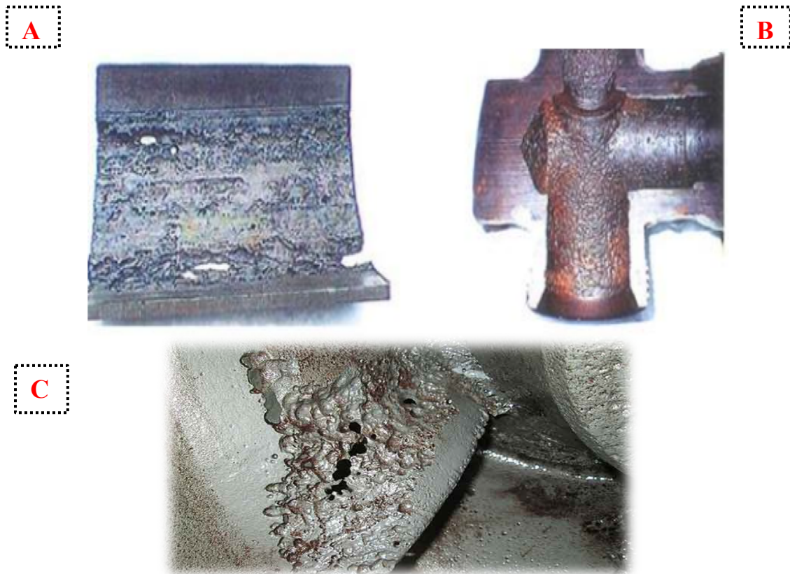
Figure 2-5: Examples of typical erosion-corrosion damage in the oil and gas industry: (A) a carbon steel pipeline, (B) a choke valve, and (C) a propeller pump [28, 6].
