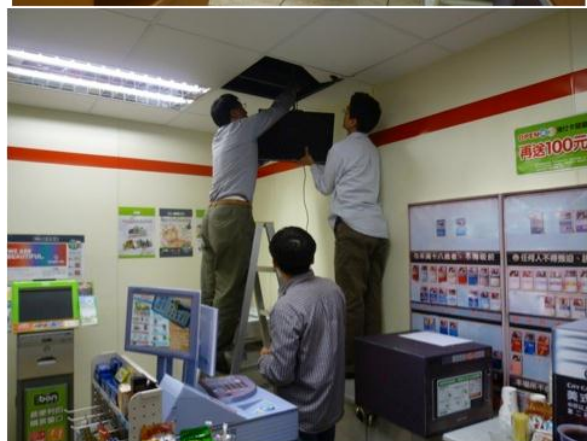
Figure 3. Sensor deployment in the CVS laboratory.
