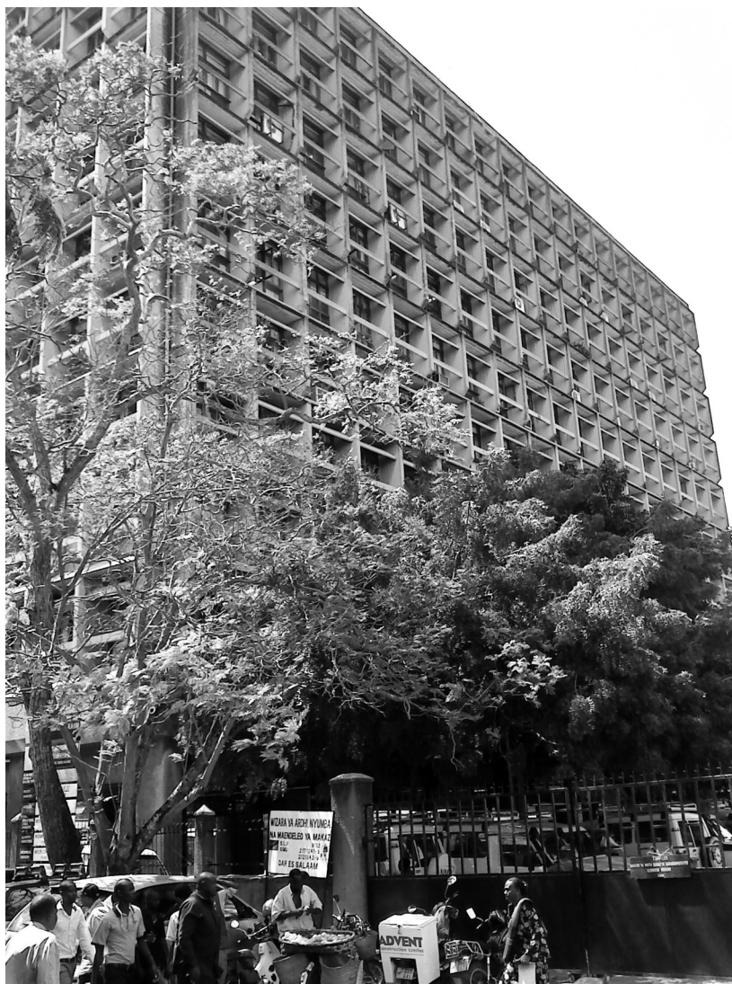
Fig 2. Ardhi House – one of the buildings poorly equipped with fire fighting means and facilities, in addition to limited awareness on the part of its users – a disaster risk!
