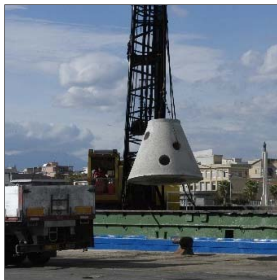
Figure 3 Installing the rocks and modules on the reef
