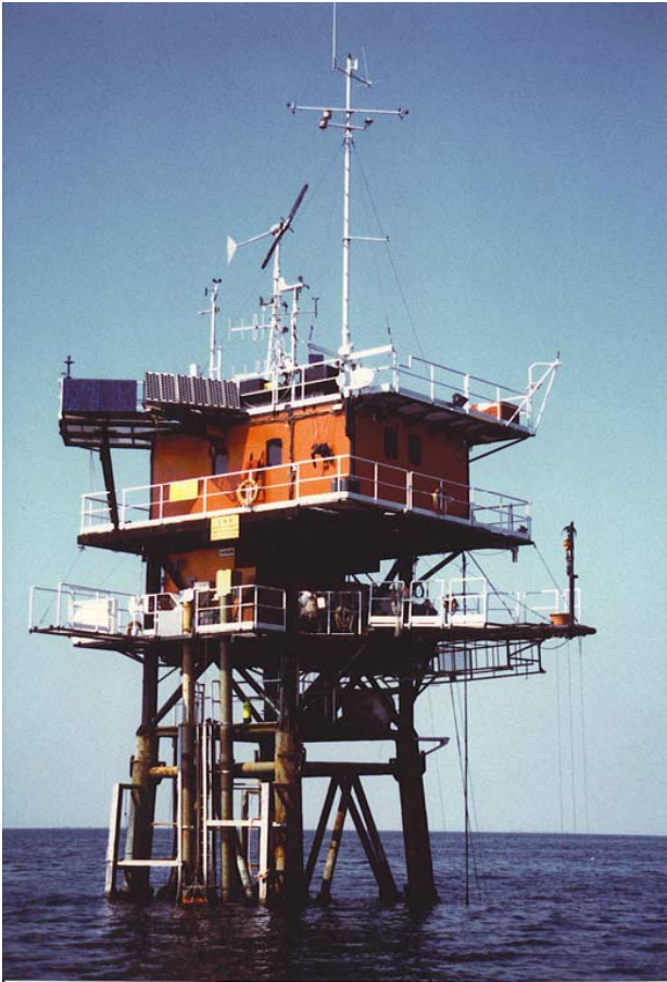
Fig. 5. The ISMAR oceanographic tower. See Fig. 2 for its position. The upper terrace is 12.5 m off the mean sea level.
