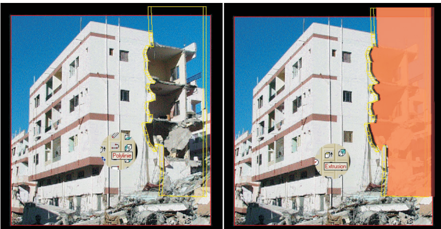
Fig. 5. Marking the run of a crack on an imported picture (original picture: Markus, 2001).
