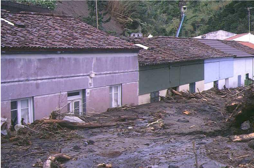
Fig. 6. Houses affected by debris flows during the 1997 Ribeira Quente event.
